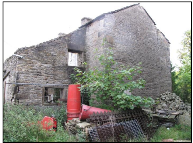
Figure 10: West Elevation Gable
