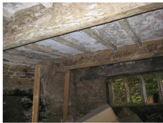
Figure 17 and 18: Existing First Floor Structure over Room 2 (there is no first floor structure over room 1 (assumed to have collapsed))
