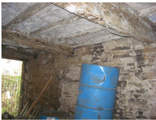
Figure 17 and 18: Existing First Floor Structure over Room 2 (there is no first floor structure over room 1 (assumed to have collapsed))
