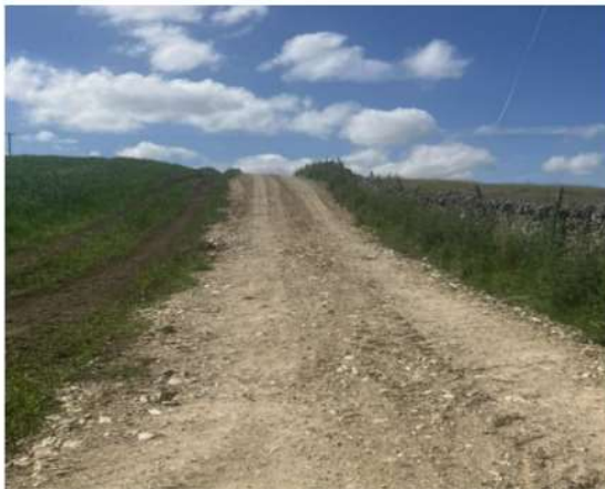
Photo 1 – Newly laid track
