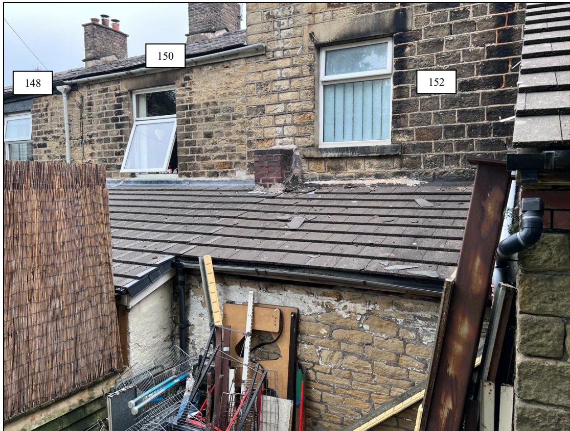
Figure 2: First Floor rear Windows of 148, 150 and 152 Station Road
