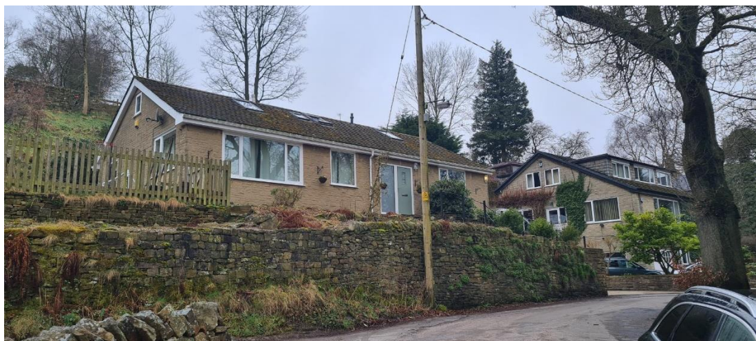
Figure 2: The property's nearest neighbour is a 2-3 storey dwelling house dating from a similar era.
