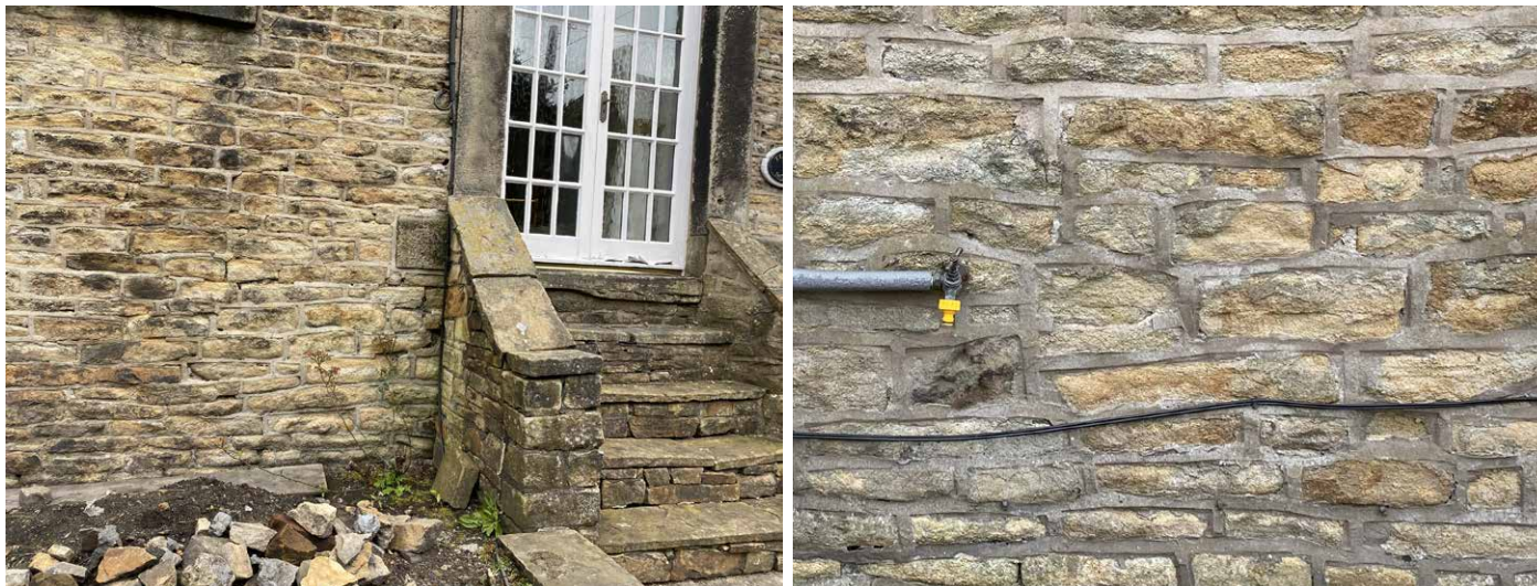
Existing random coursed gritstone walls with cement strap pointing.
