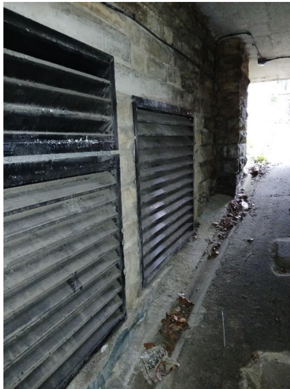
Figure 3 – Louvred openings in the façade, leading to the basement plant room
