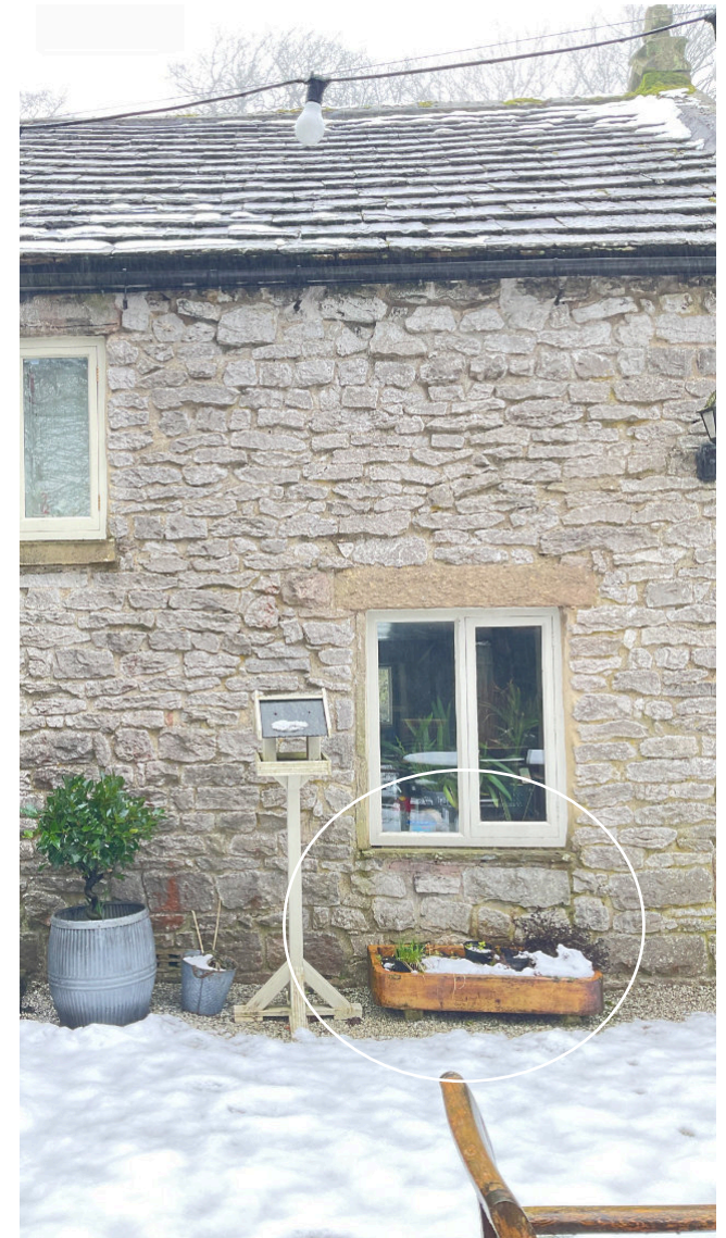
Fig. 1. Above: Existing north garden wall elevation.
