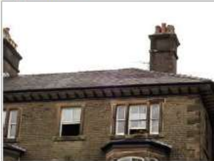
Front of roof
