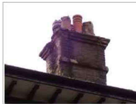
Left side of chimney
