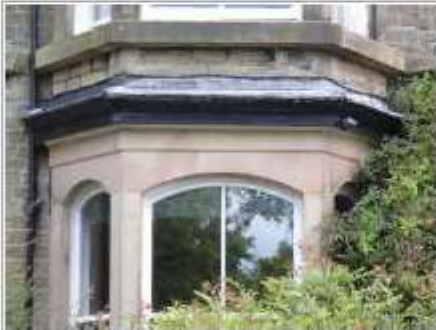
Left bay roof
