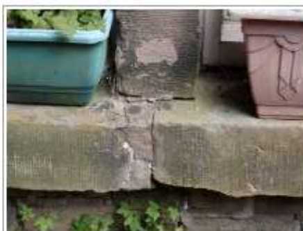
Eroded stonework
