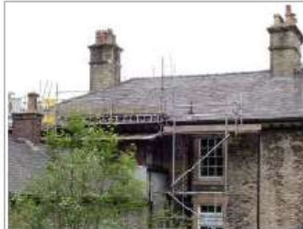
Rear of roof
