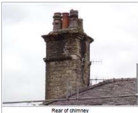
Rear of chimney
