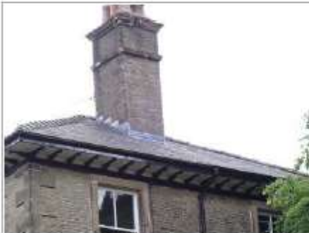
Right gable roof
