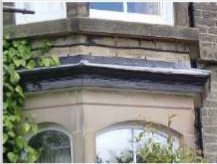
Right bay roof
