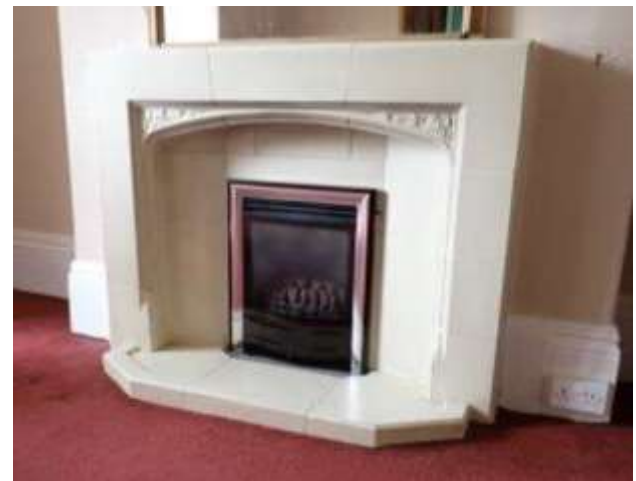
2. Existing fireplace with a coal-effect gas fire fitted
