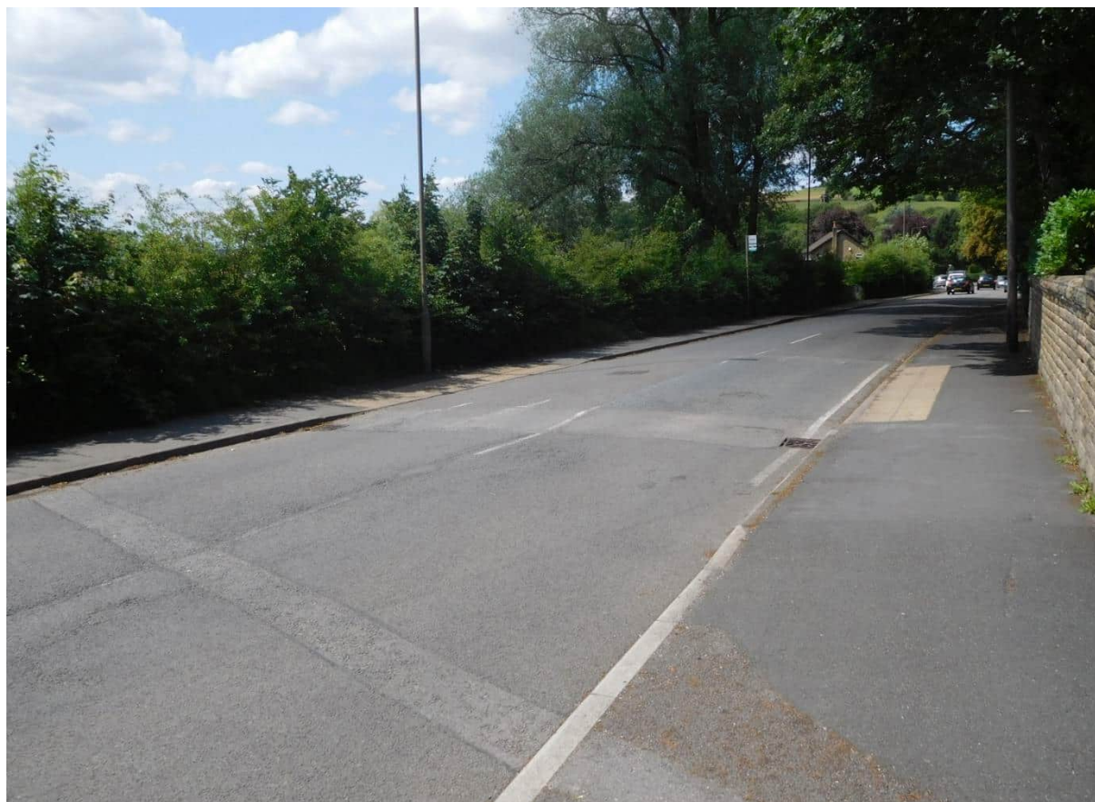
Figure F: Tactile Paving and Dropped Kerb Crossing Point on Talbot Road
