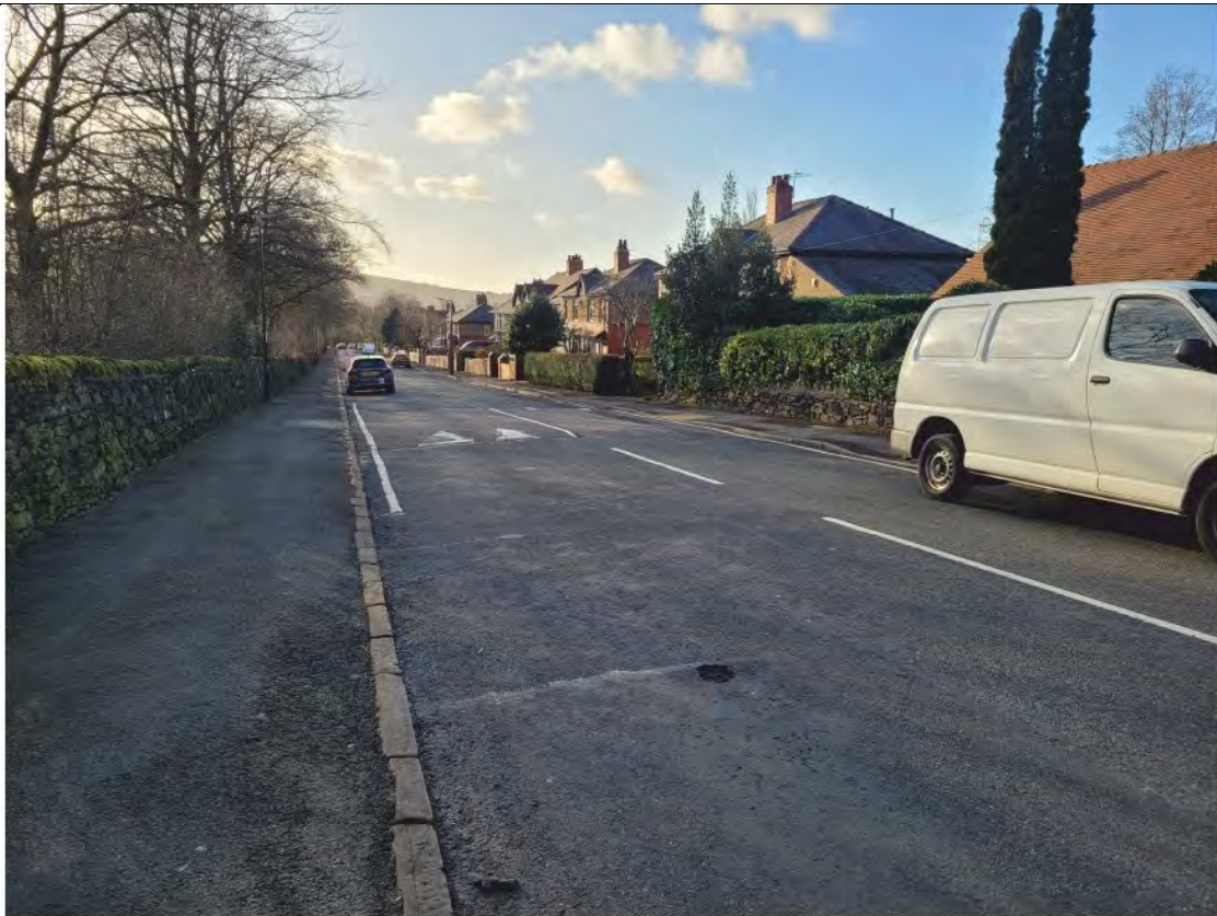
Pl. 15 Fauvel Road looking south-west. Norfolk Square Conservation Area west boundary to left
