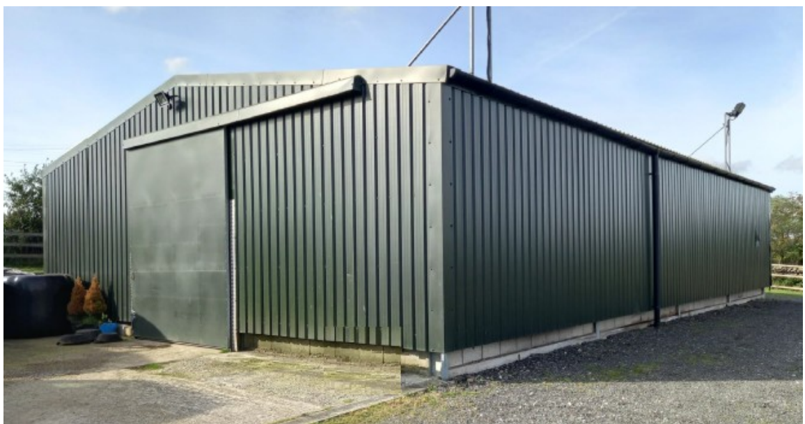
Figure 3: View of the Building
