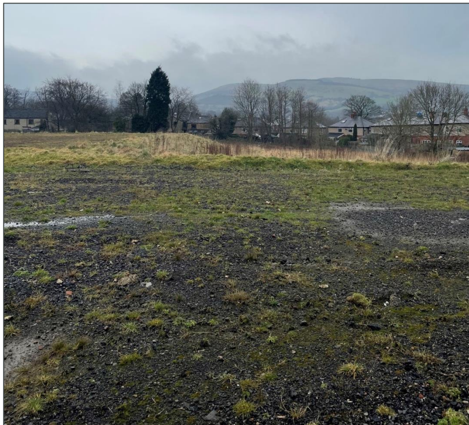
Figure 12: School site post-demolition
