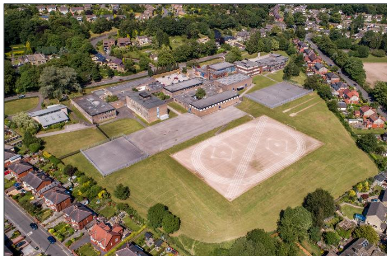
Figure 9: School site prior to demolition
