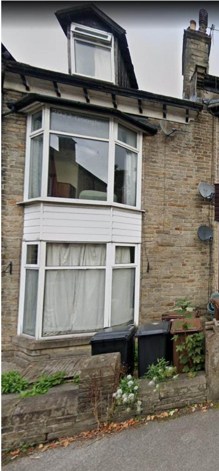
54 West Road showing White UPVC Windows
