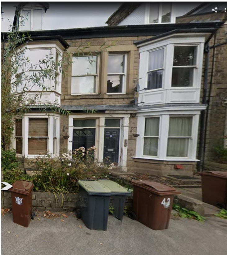
48 WEST ROAD SHOWING THE EXISTING TIMBER WINDOWS IN THE APPLICANT DWELLING
