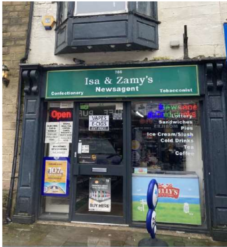
Above: Replacement unauthorised shopfront
