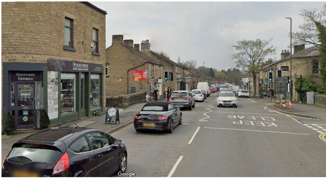
Fig 1: (APPENDIX A) Street View Photo of the Appeal site on the gable of 117 High Street West Glossop SK13 8BB showing the non-illuminated advertising sign viewed in a predominantly commercial street scene
