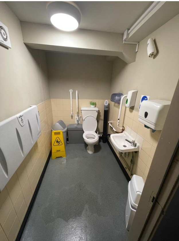
Existing Accessible Toilet
