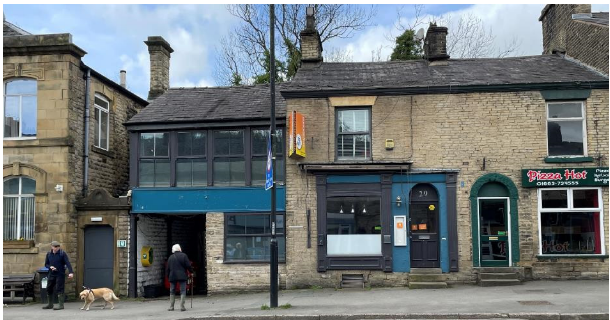
Front of property facing Market Street
