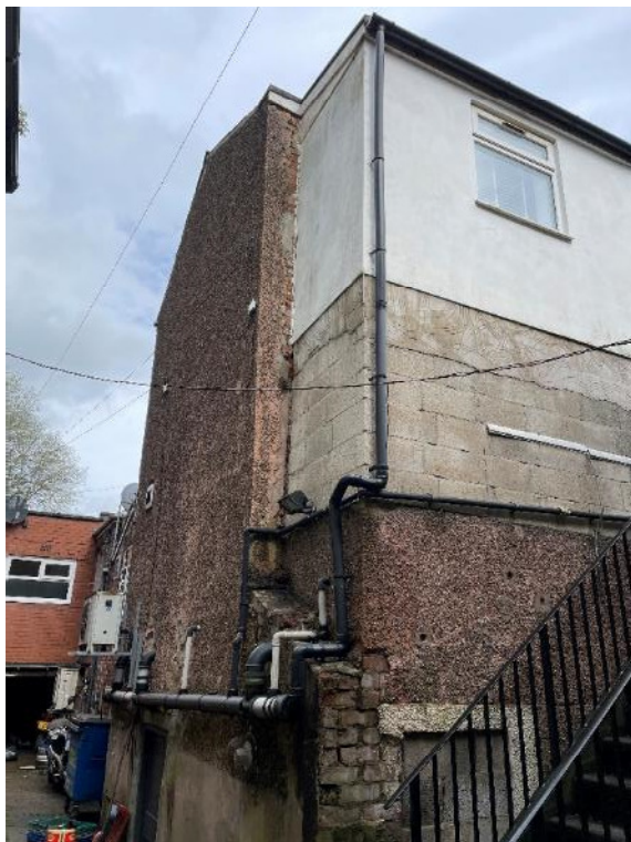
Rear of building showing bay window extension
