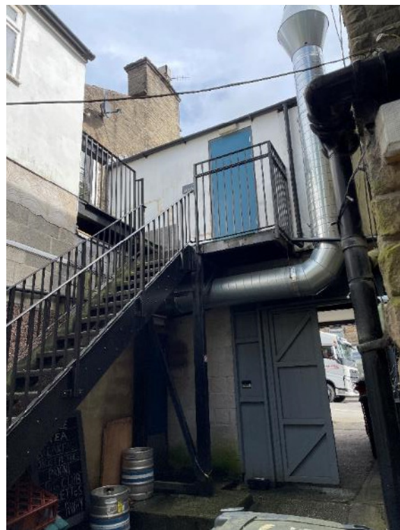
Rear of building showing fire escape and access to first floor flat
