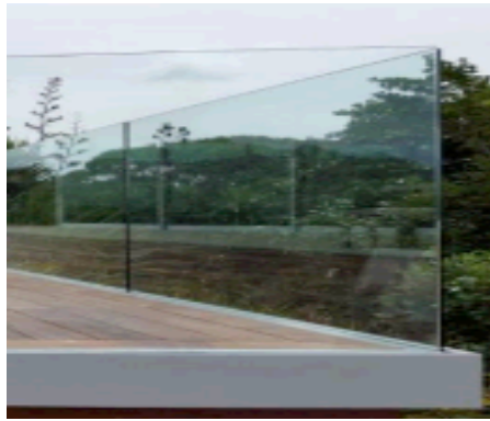
Example of Frameless Glass Balustrade System to Decking
