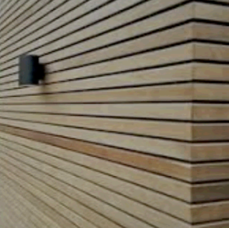
Example of Timber Cladding to Raised Decking walls
