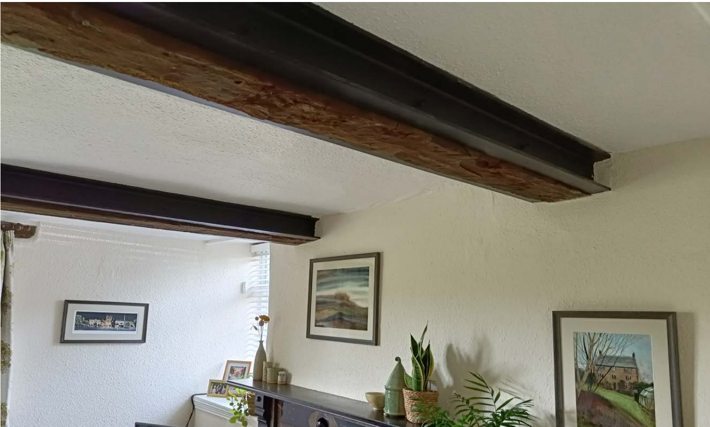
Figure 18 Beams 7 and 8 already flitched
