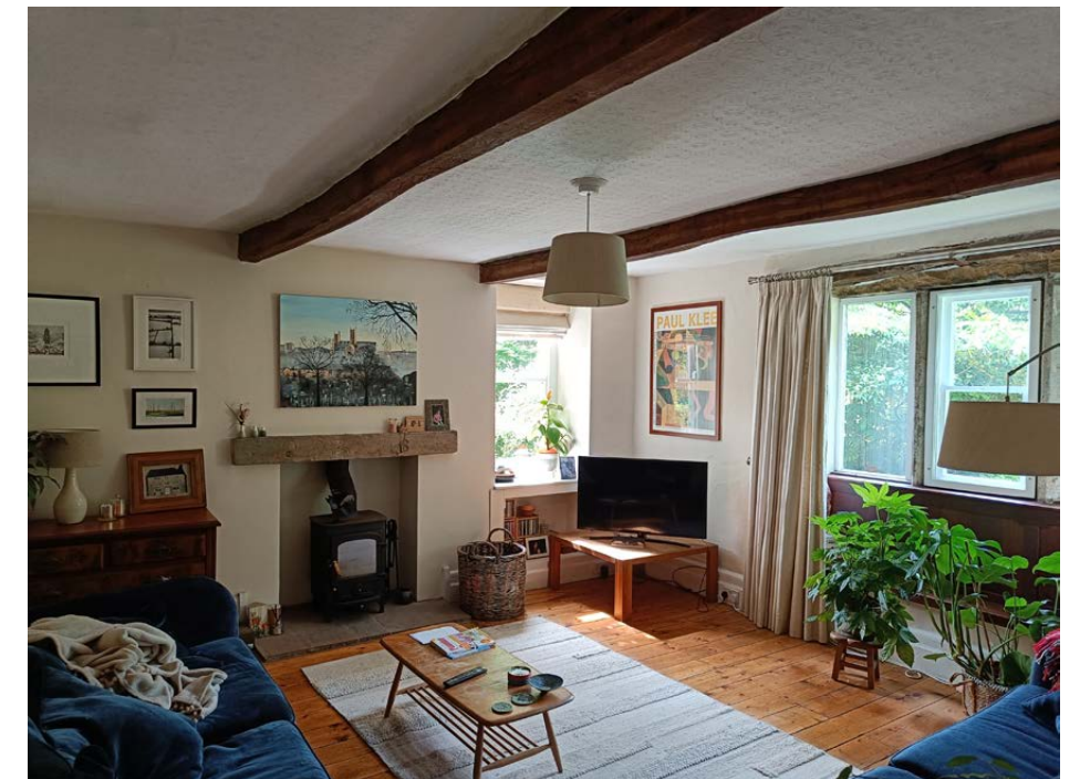
Figure 21 Beam 3 (nearest window) proposed to be flitched
