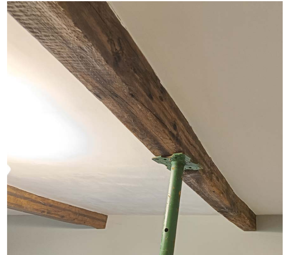
Figure 20 Beams 1 and 2 proposed to be flitched
