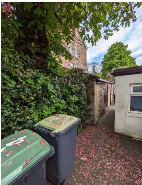
Figure 6 Rear of Unit 1 from Cresswell Street
