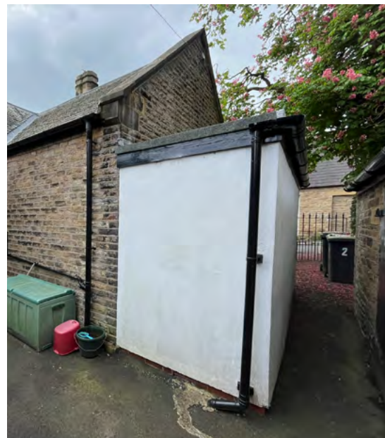
Figure 7 Rear of Unit 1 toward Cresswell Street
