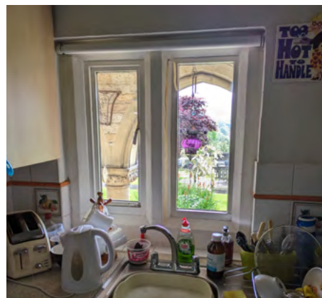
Figure 3 Example of painted stone surround
