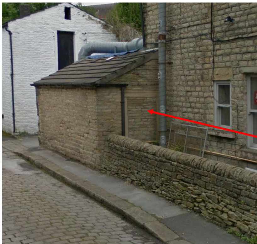
Existing 'blocked-up' opening – location of proposed entrance on front elevation.
