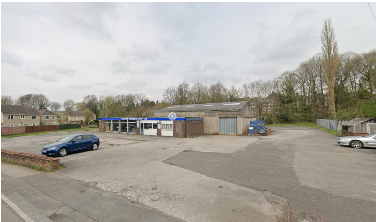
The application site
