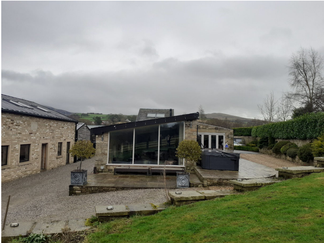
Figure 1 – western elevation of house as existing.
