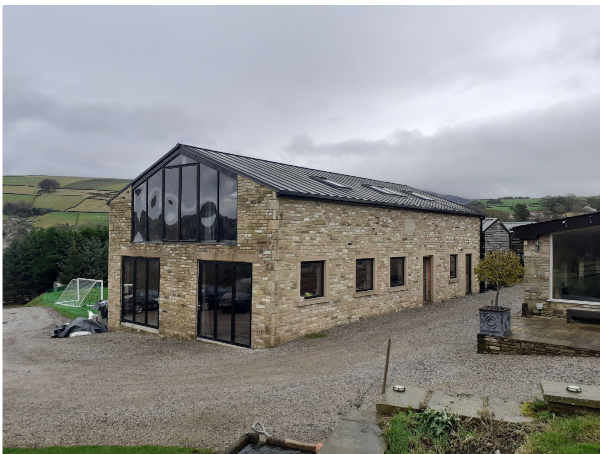
Figure 3 – Barn as existing
