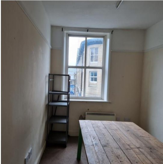
Figure 4: The First Floor and a narrow office exemplifying the non-original layout of the First Floor.
