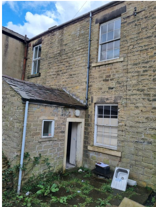
Figure 3: Existing rear elevation of 8 Henry Street access via a parking area off Railway Street.
