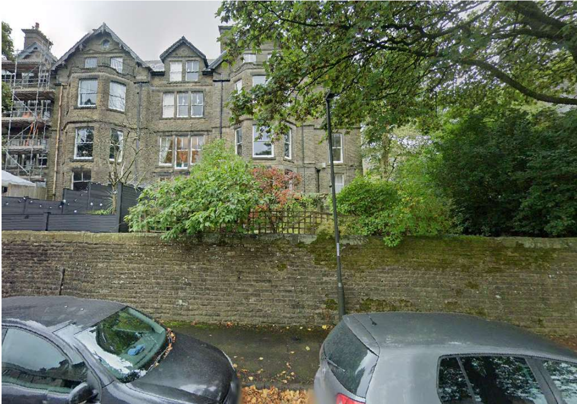
Figure 1 – google street view of the application site as viewed from Hartington Rd.
