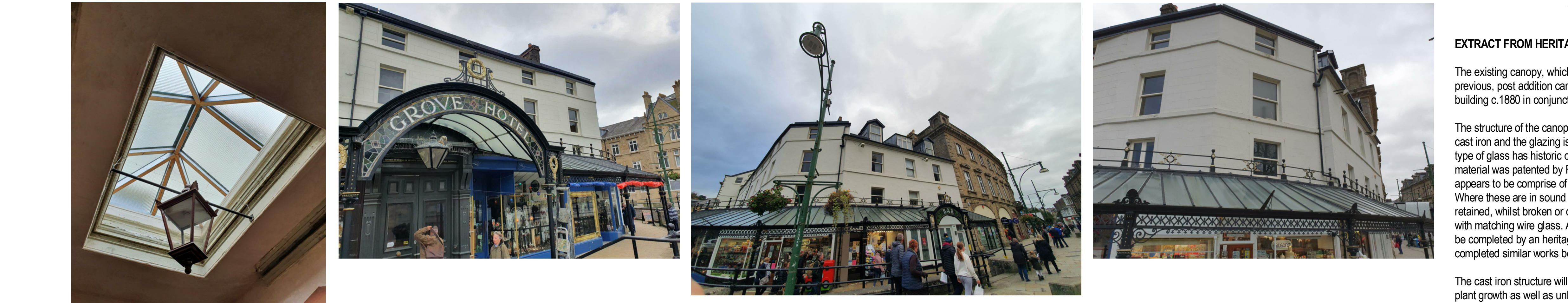
6. View: Internal US of roof lantern within main entrance lobby - to be replaced (design to match existing lantern) 7. View: View: Stained glass signage over main entrance 8. View: Stained glass signage "BAR" - missing and damaged panels to be replaced 9. View: Top of glass canopy looking towards Spring Gardens - indicating existing condition of paintwork and damaged glass panels - paint work to be made good (colours to match existing)/glass panels to be replaced with Georgian wired glass (to match existing)
