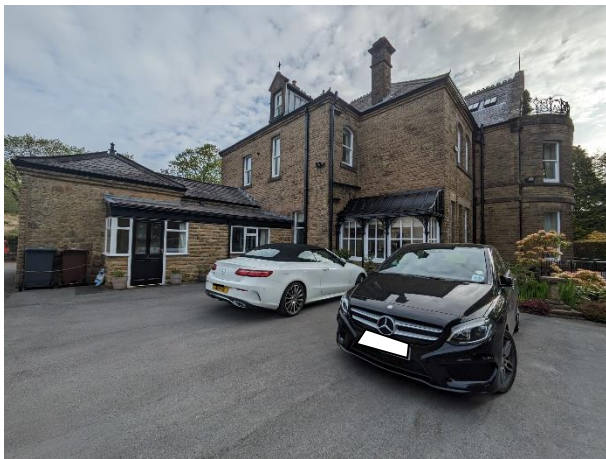
Fig 1: Infilled porch seen from within car park to west
