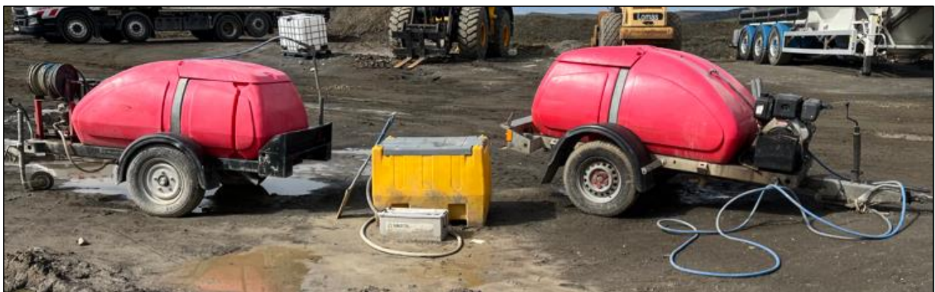
Image 1: A photograph of the Wheel washing facilities on site
