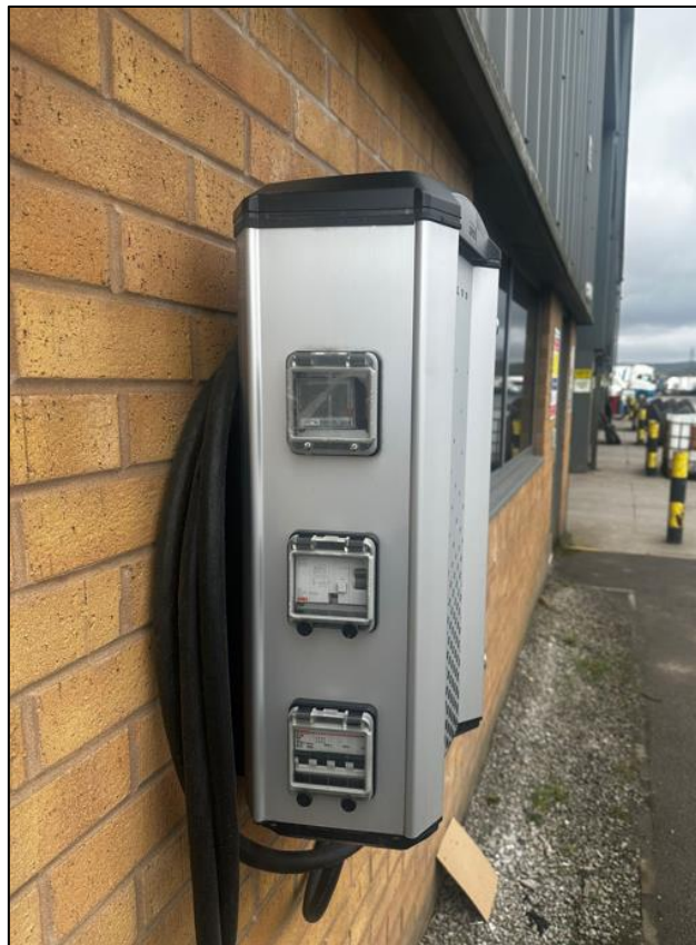
Image 3: Photograph of the HGV wall-mounted charging point at the main office at Lomas Distribution
