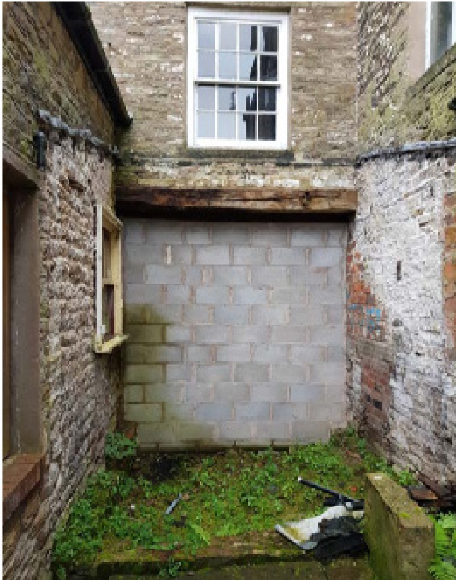
Courtyard with entrance into bar blocked up.
