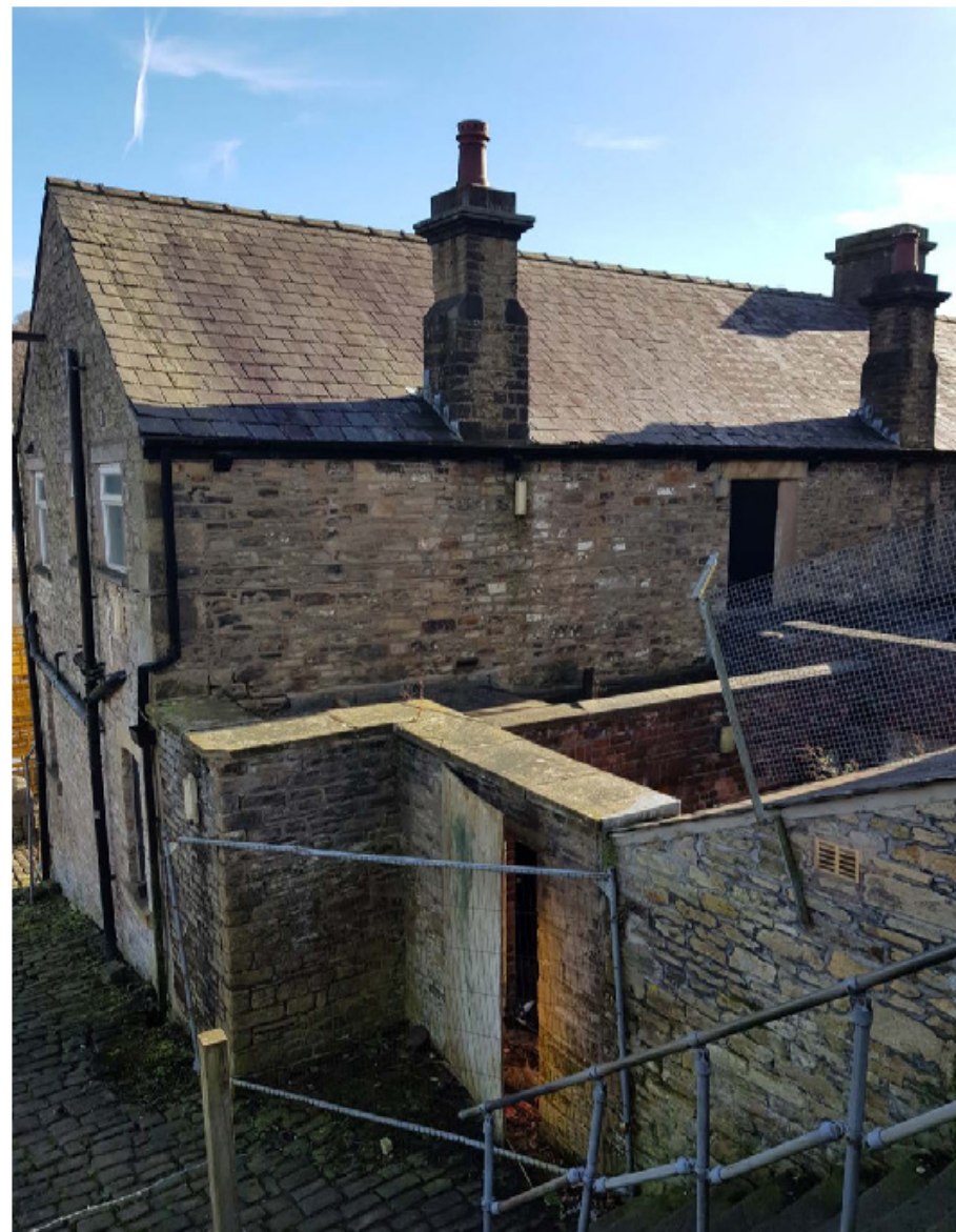
View of North gable from public footpath.
