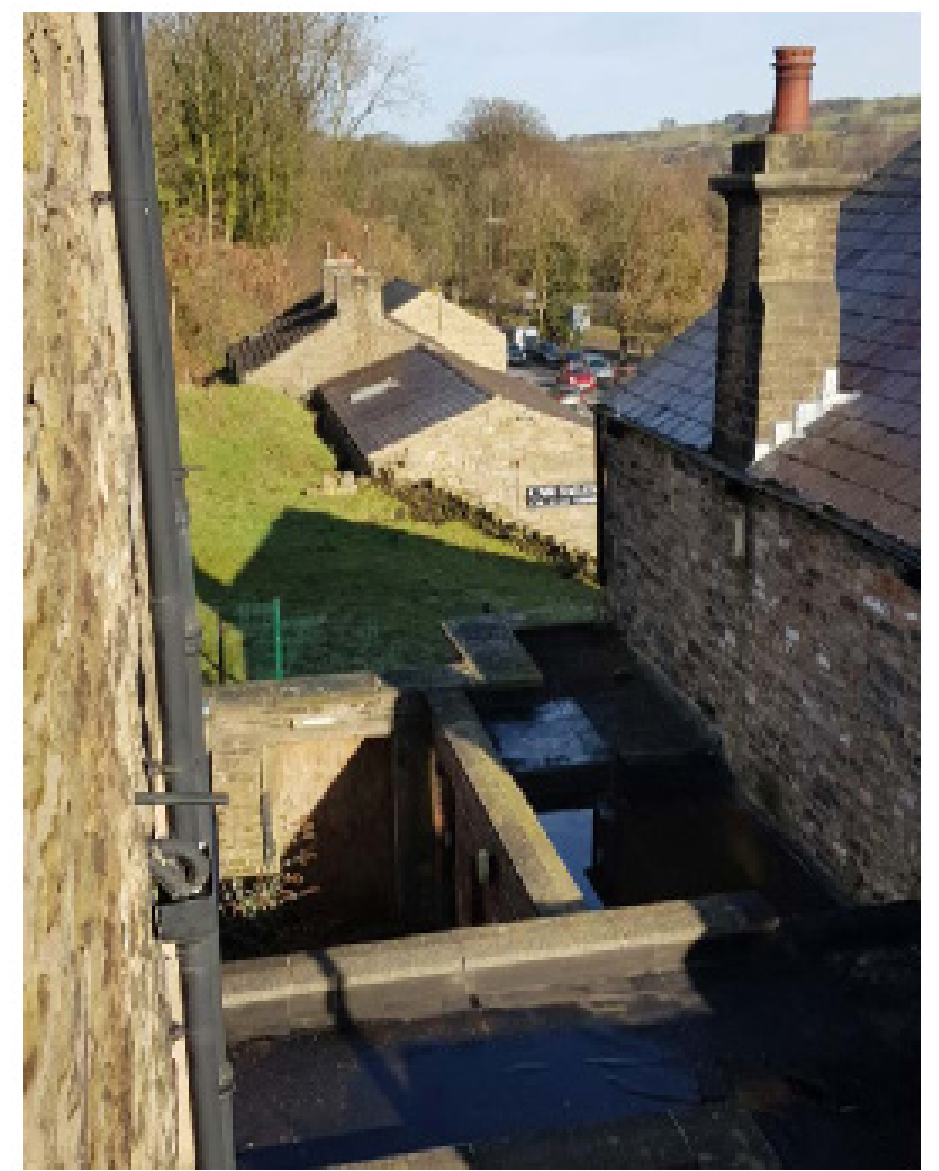
View of courtyard from second floor window
