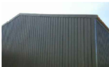
Example of profiled vertical wall cladding
