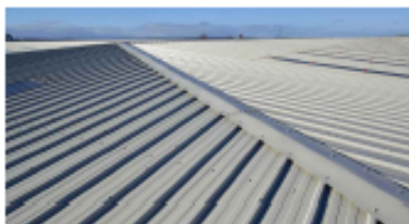
Example of profiled roof sheeting
