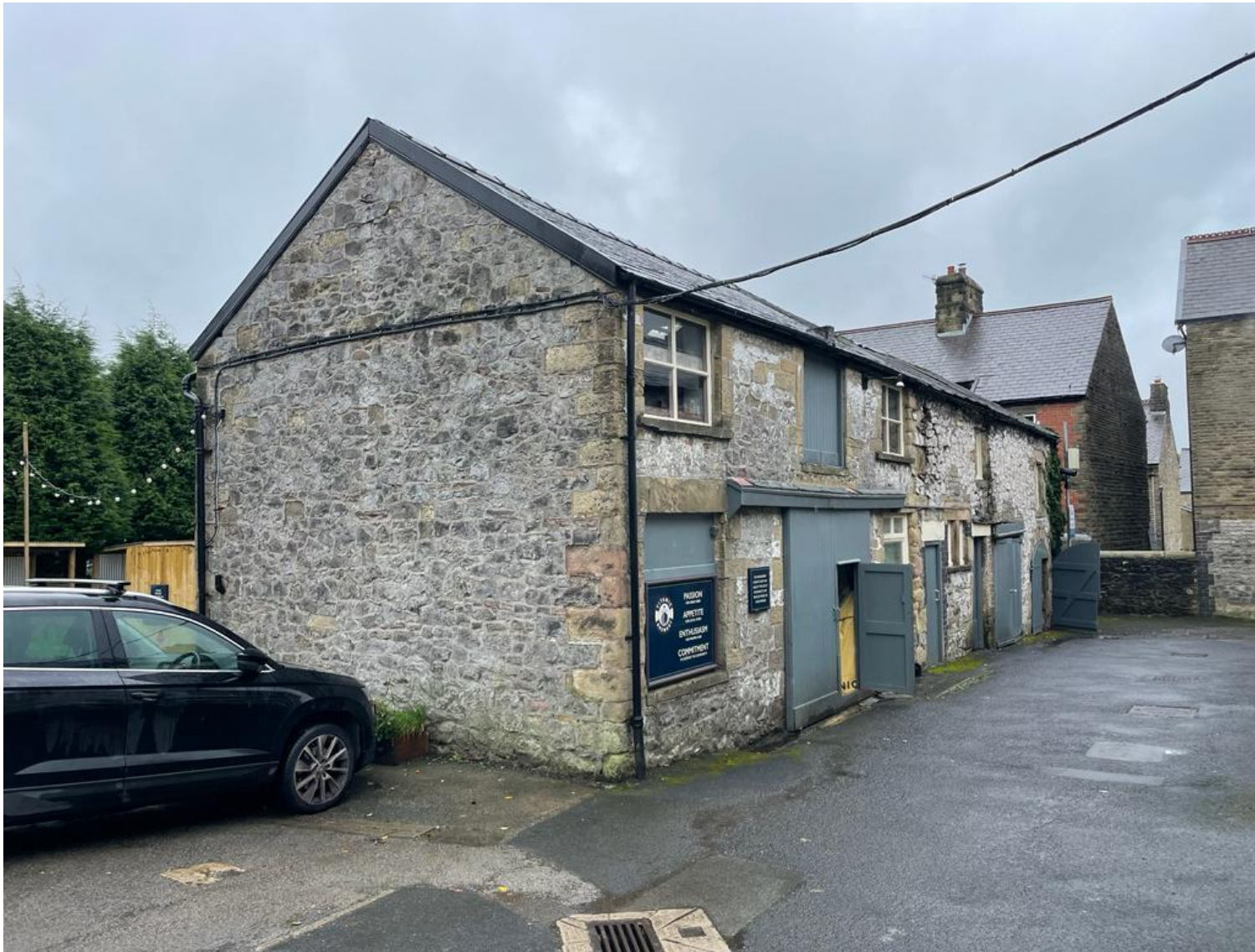
View of NW gable and front elevation of Out-building.
