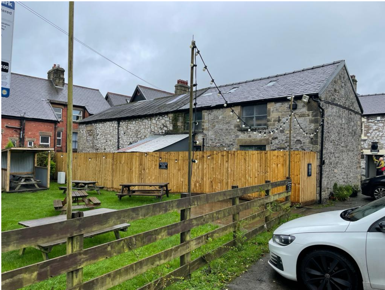
Rear of Out-building – showing part corrugated sheet roofing.
