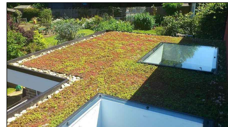
SEDUM ROOF COVERINGS WITH FLAT GLAZED ROOFLIGHTS
