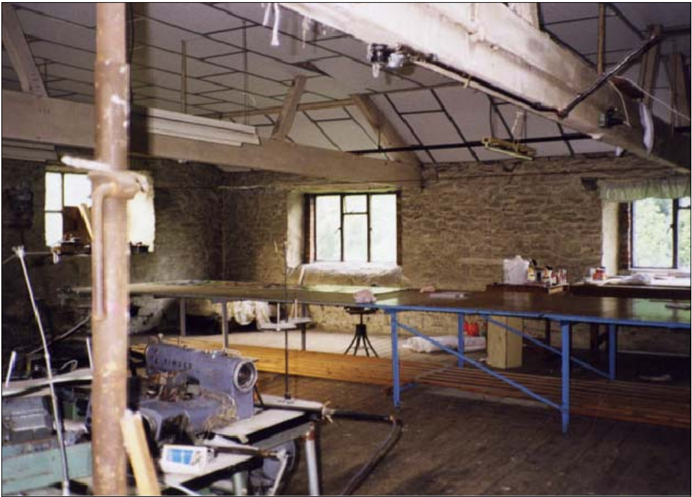
Photo 3. Internal photo showing windows from the upper floor. The brick work suggests these aren't original windows, potentially mid 20th century. Side hung casements with a central top hung fan light. The windows to the left look older and suggest the windows were broken up with a central transom
