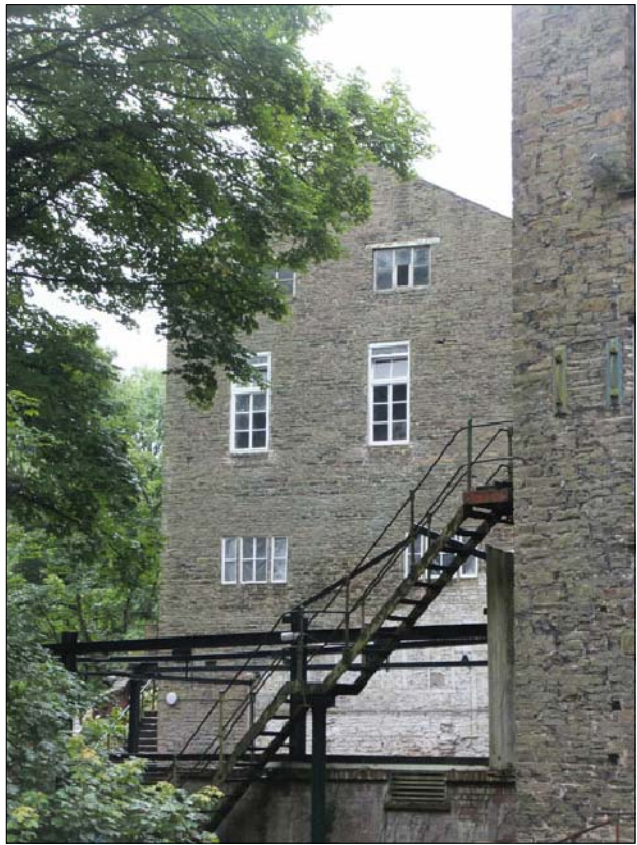
Photo 1. Showing inward opening windows on upper floor.
