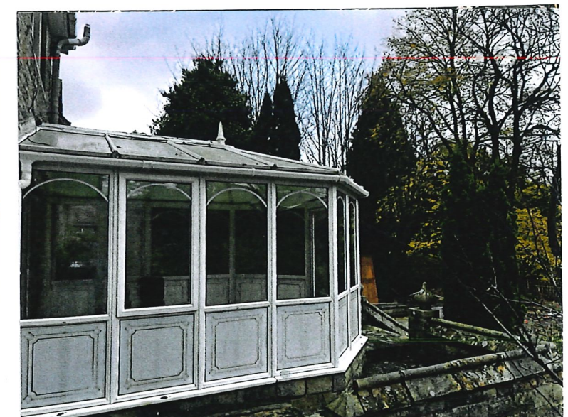
VIEW LOOKING SOUTH EAST
