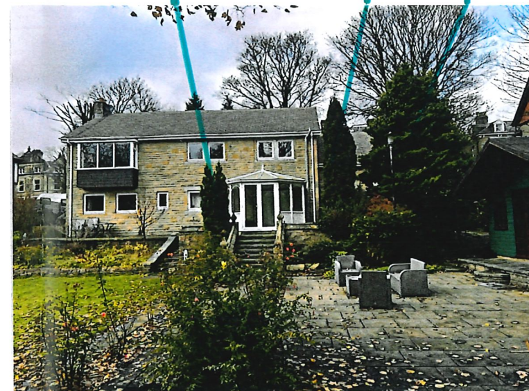
VIEW LOOKING NORTH
