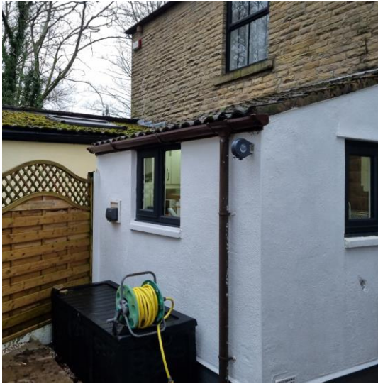
Figure 3: Existing single storey part of dwelling to be demolished.
