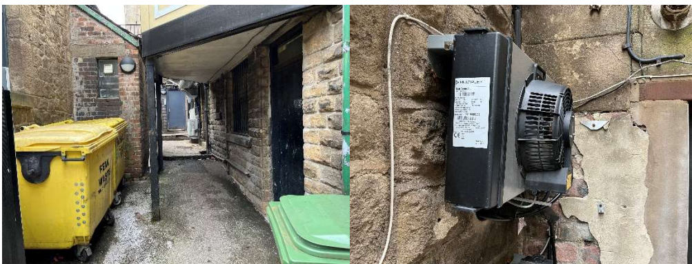
Rear yard and Walkthrough
