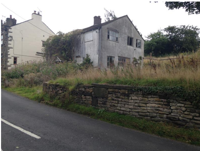
Photo 2: View from Town Lane towards derelict cottage, illustrating poor quality later extension.
