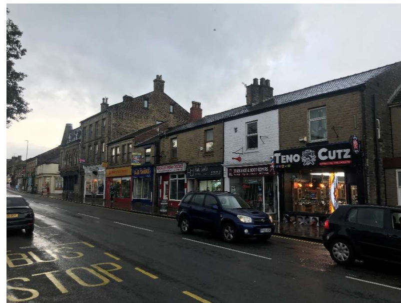
View looking South West towards no.81 High Street West
