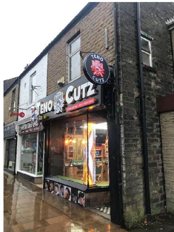
View Looking towards no.81 High Street West
