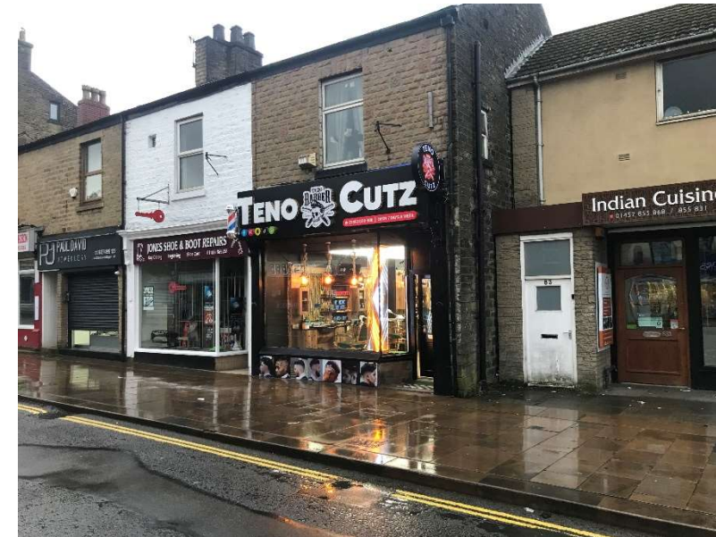
View Looking from no.83 High Street West
