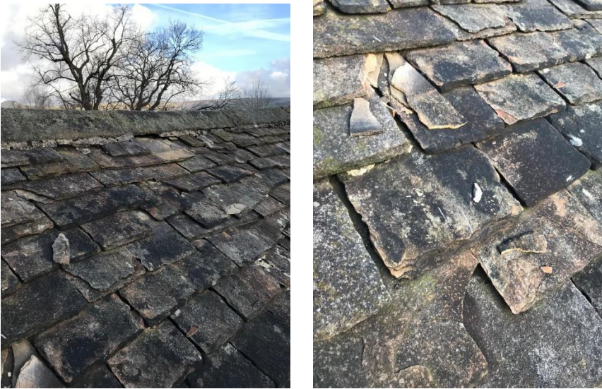
External Images of Stone Roof Condition
