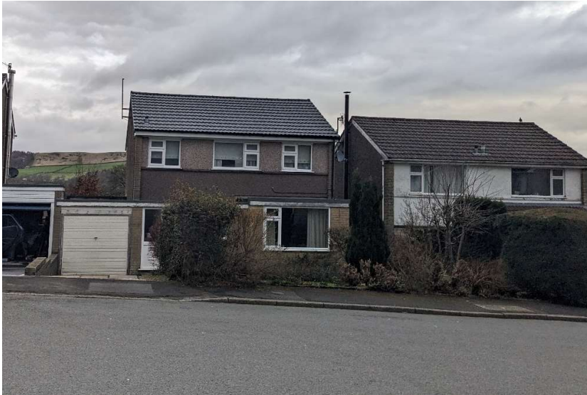
Figure 4 – Image showing flat roof front extension at no. 12 Arbore Grove.
