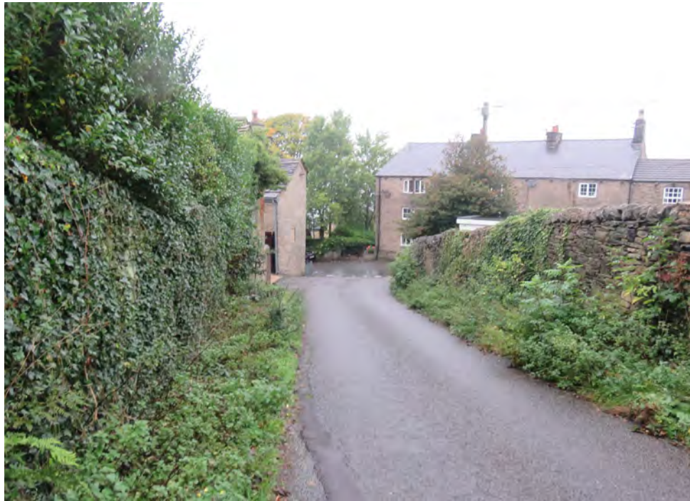
View looking North down Chapel Brow.
