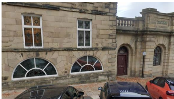
Figure 5: Arched windows to the Natural Mineral Baths building.
