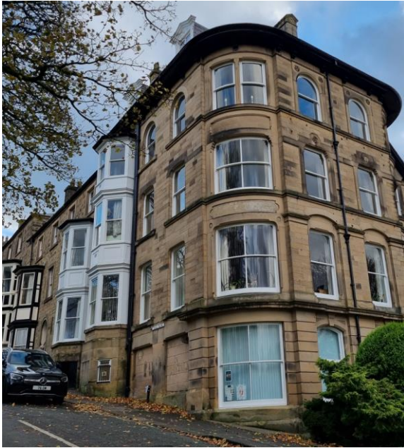
Figure 7: View from junction of Hall Bank and Hartington Road looking up Hall Bank. The window to the base of the bay nearest the camera has a steel security grille.
