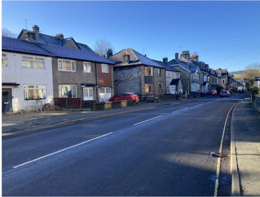
Fig 2: Site as existing in 2024 with wall demolished
