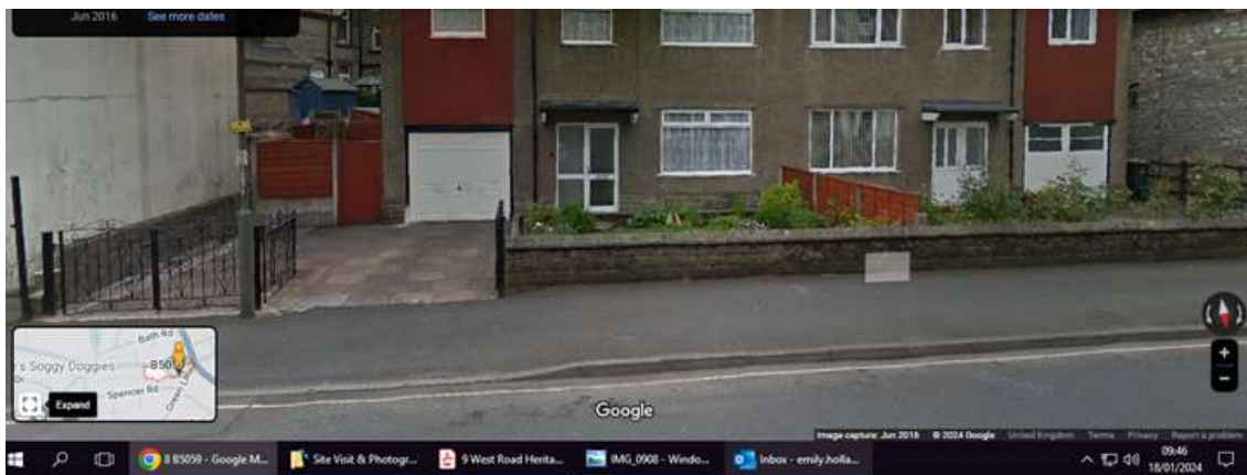
Fig 1: Boundary Wall and access as existed in 2016
