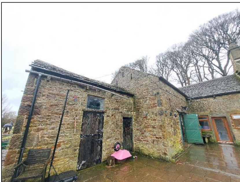
Photograph 1 showing south facing elevation of the barn
