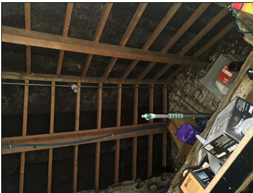
Photograph 14 showing the underside of the roof in the storage section of the barn
