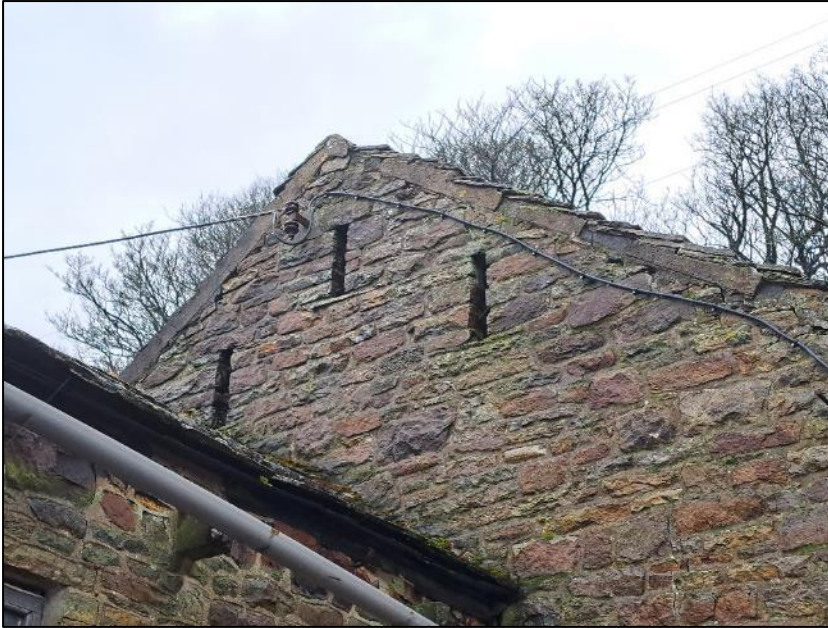
Photograph 3 showing vents on the west facing elevation
