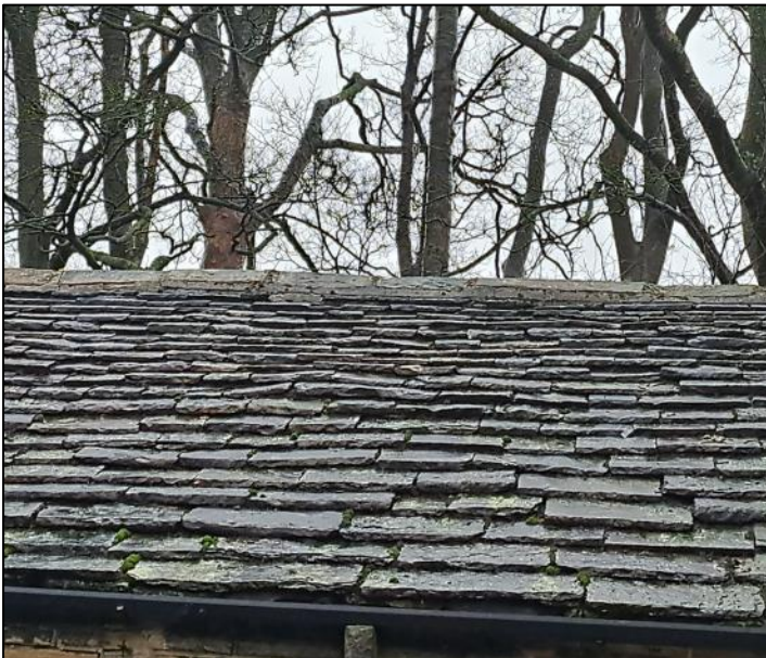
Photograph 4 showing a section of the roof
