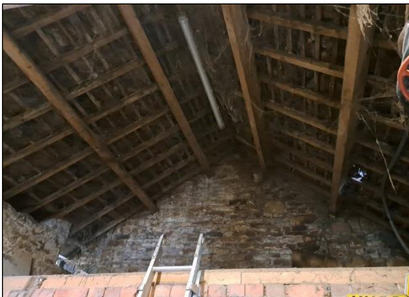
Photograph 8 showing the underside of the roof of the barn
