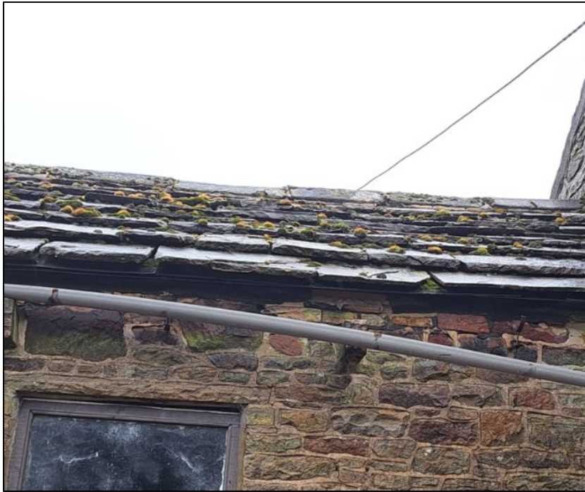
Photograph 5 showing a section of the roof
