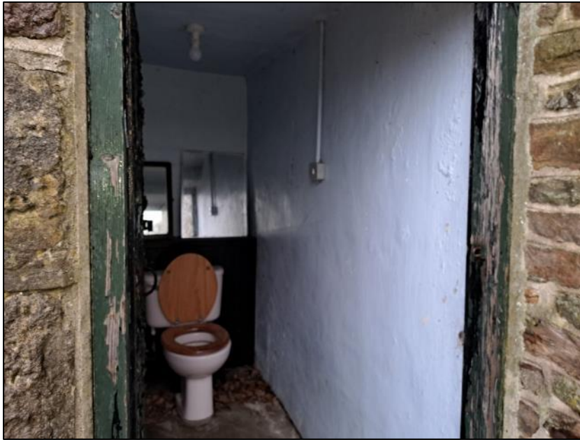
Photograph 13 showing an interior room
