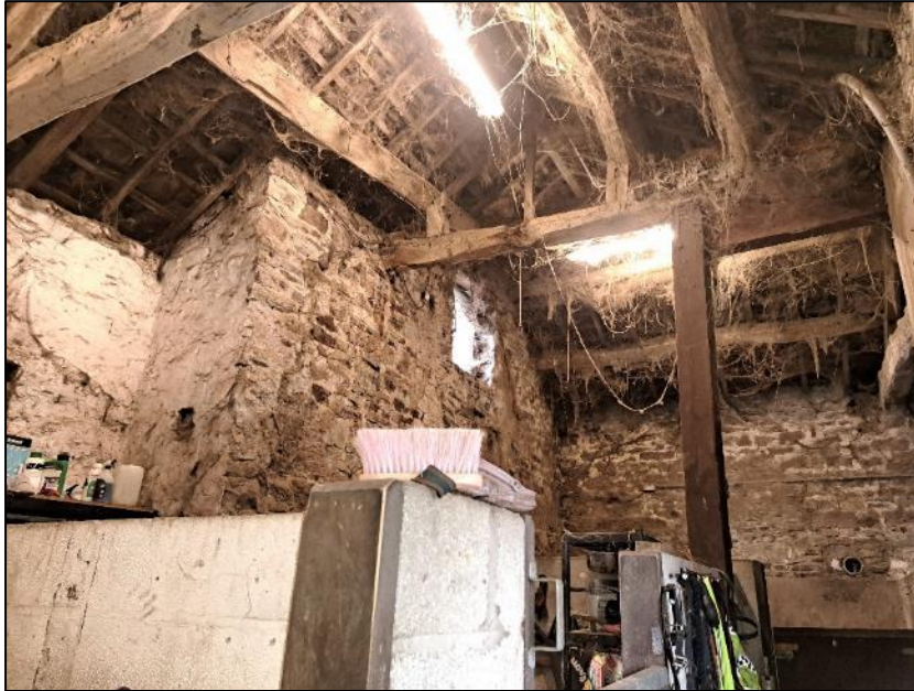
Photograph 7 showing the interior of the stable section of the barn
