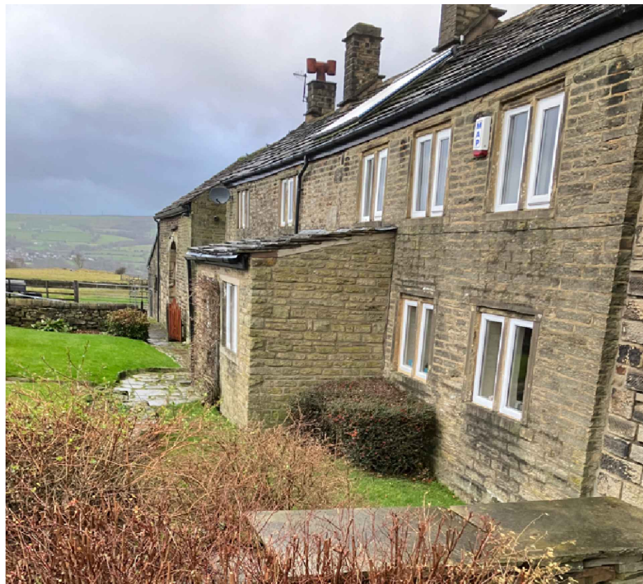
2. Elevation photograph from east showing storm porch
