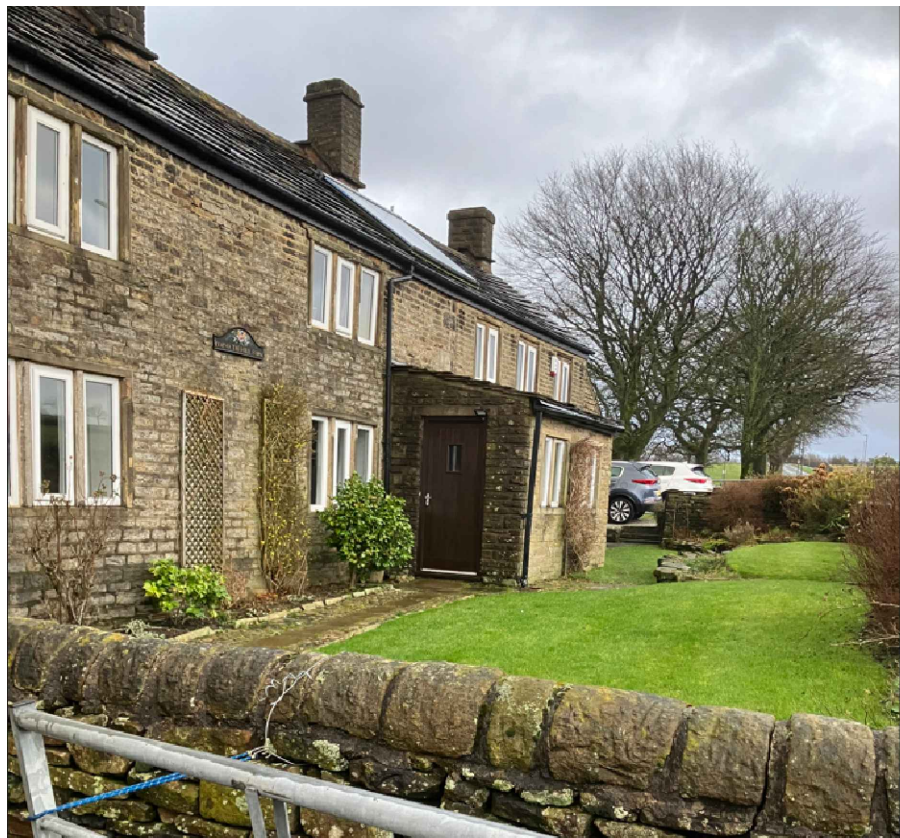
1. Elevation photograph from west showing storm porch and existing front door
