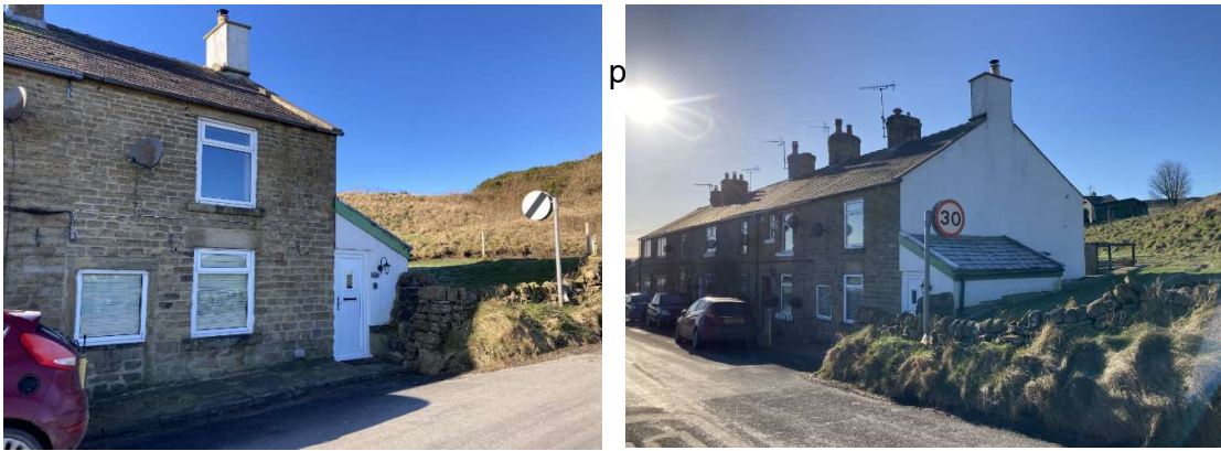
Above: Photographs showing the principal and side elevation of No.67 Meadow Lane and its relationship with elevated grass land beyond.
