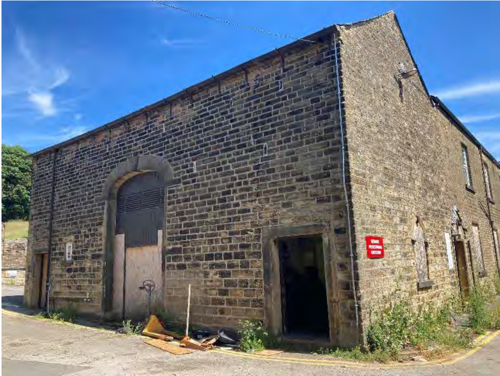
Plate 5. View of the west facing elevation of the Barn
