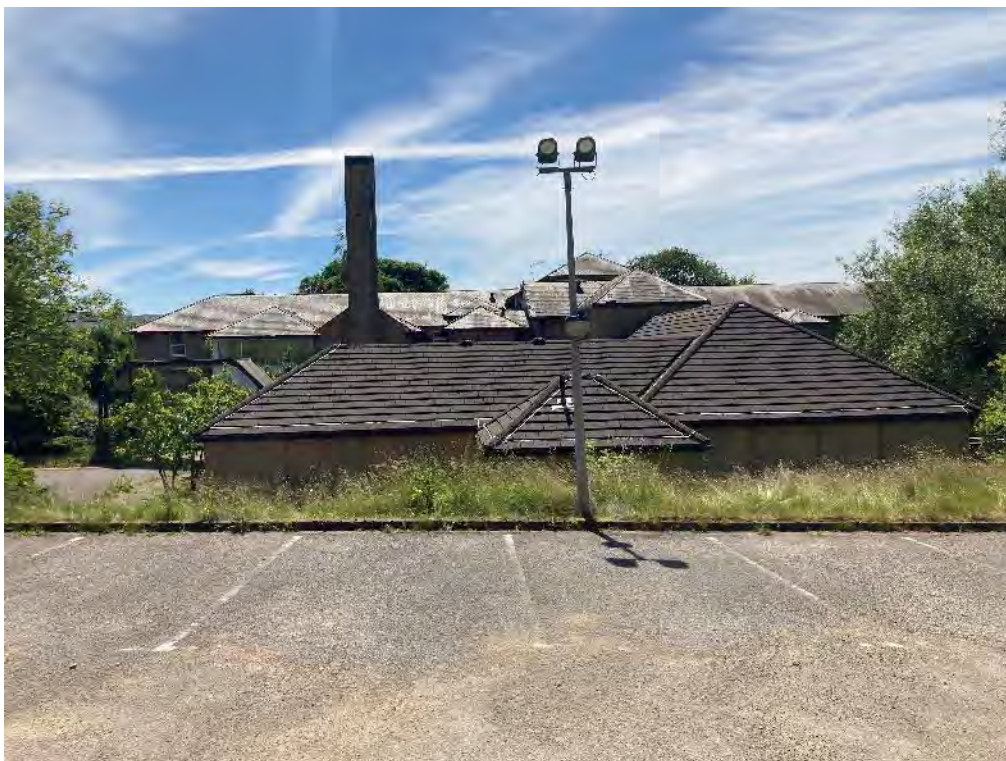
Plate 6. View from the rear car park towards the rear of the Ward Block.
