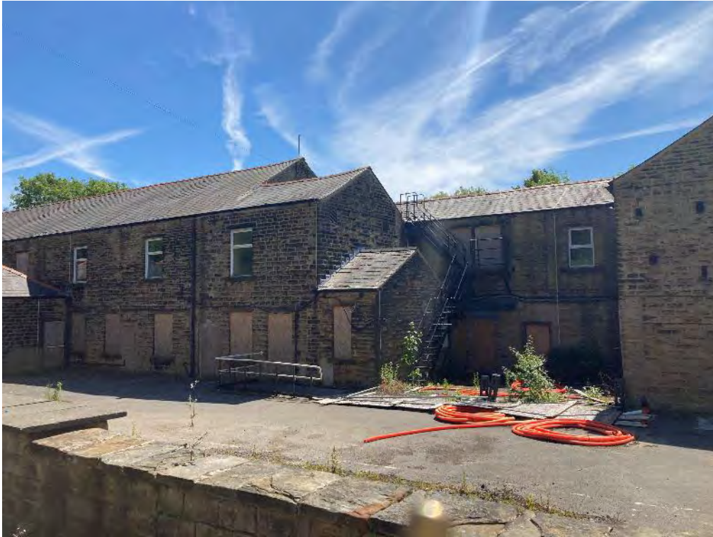
Plate 3. View of the north facing (rear) elevation of the Administration Block, showing the single pile infill block between the main block (left) and the Barn (right)
