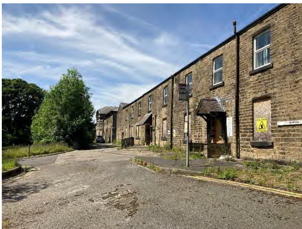
Plate 2. View westwards along the principal south facing elevations of the Administration Block and the Ward Block
