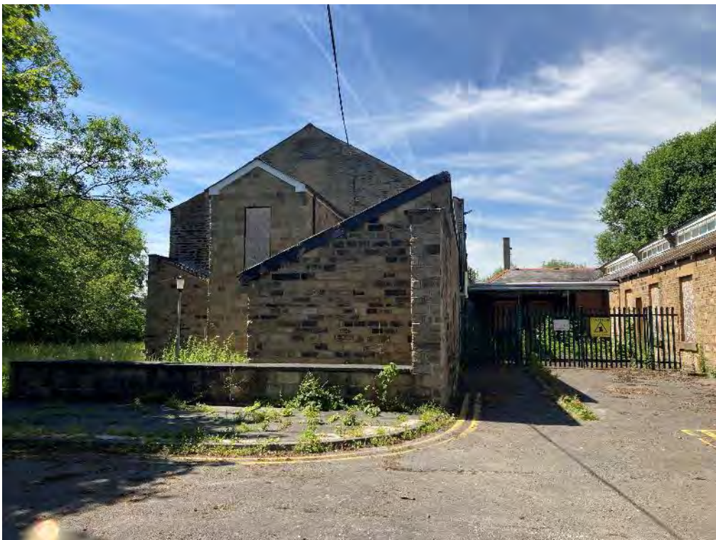
Plate 4. View of the east end of the Administration Block and ancillary extensions, with the Kitchen and Mortuary to the rear (right)
