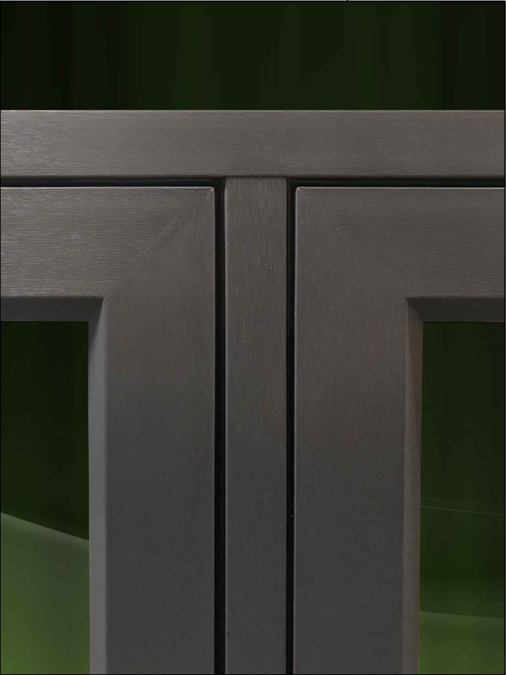
WINDOWS ARE REHAU 'RIO' FLUSH CASEMENT WINDOWS IN ANTHRACITE GRAIN. RECESSED 100mm FROM RENDER FACE
